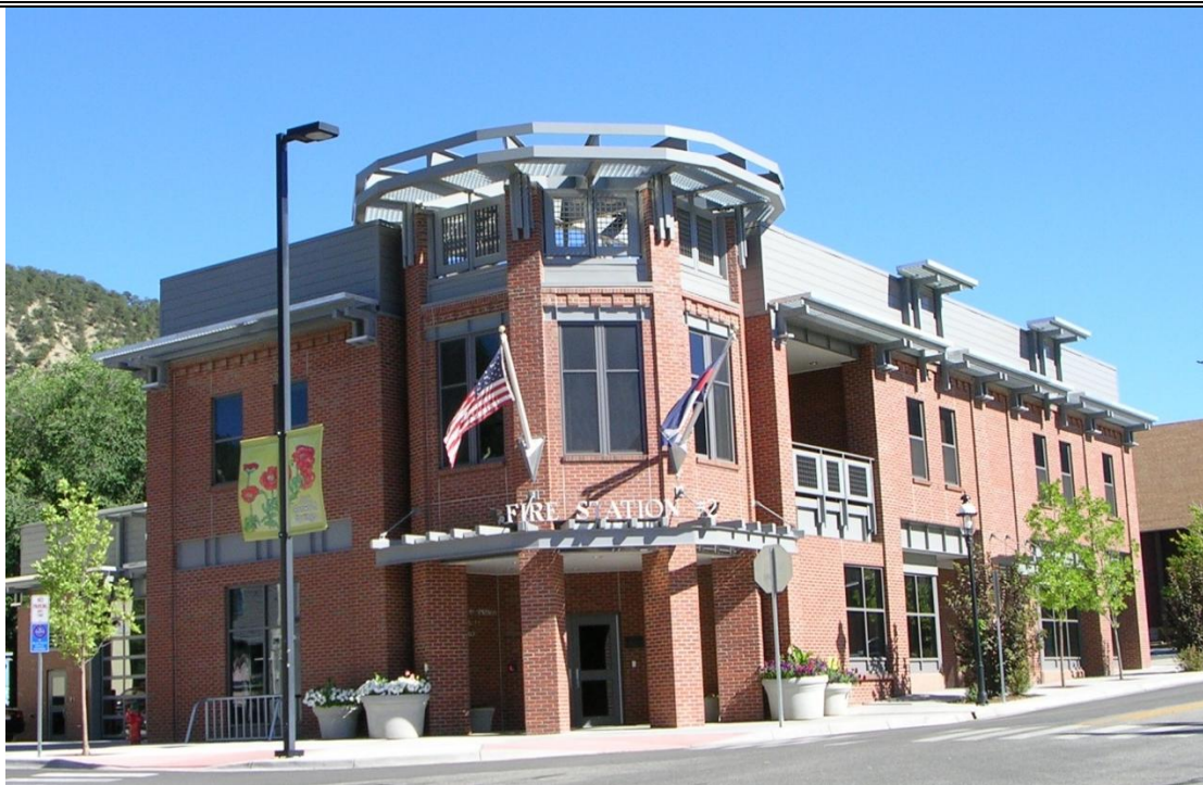
Figure 10: GSFD Fire Station No. 72 (2) Address: 806 Cooper Avenue, Glenwood Springs, Colorado 81601
