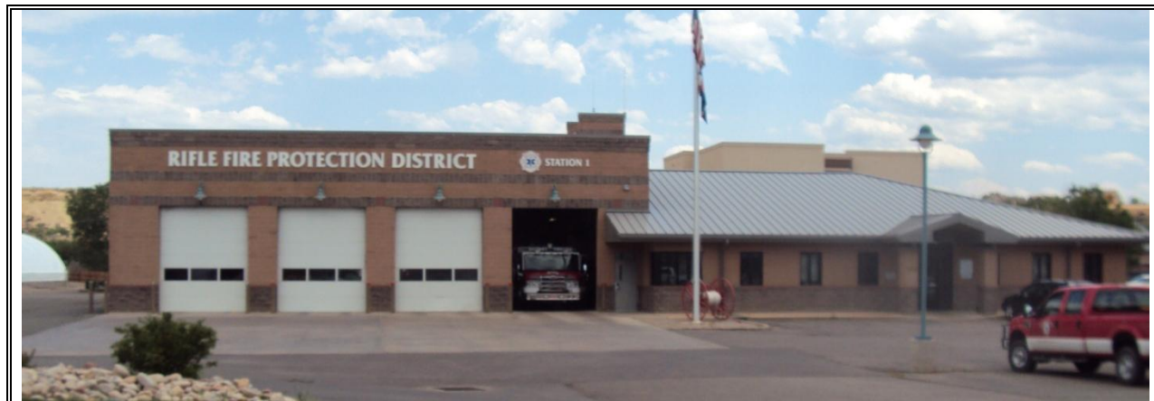
Figure 12: RFPD Fire Station No. 41 (1) Address: 1850 Railroad Avenue, Rifle, Colorado 81650
