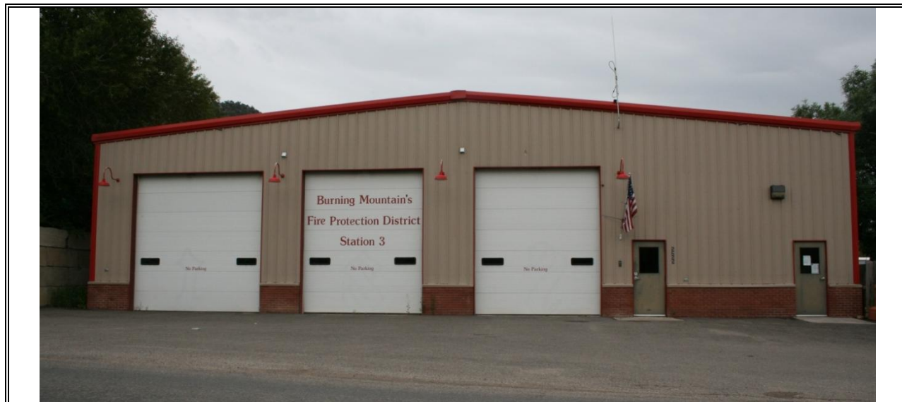
Figure 7: BMFPD Fire Station No. 63 (3) Address: 5255 County Road 335, New Castle, Colorado 81647
