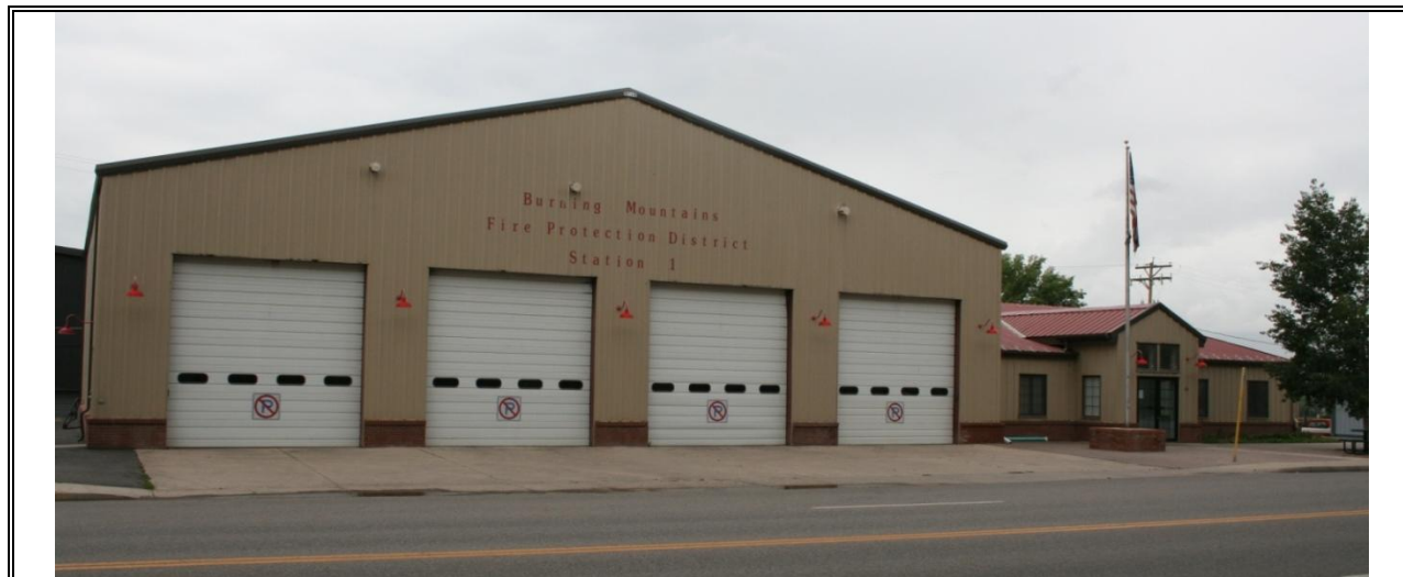
Figure 5: BMFPD Fire Station No. 61 (1) and Administration Address: 611 Main Street, Silt, Colorado 81652
